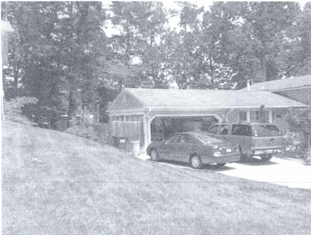
Picture 2: Left, front view of the garage taken July 2011
