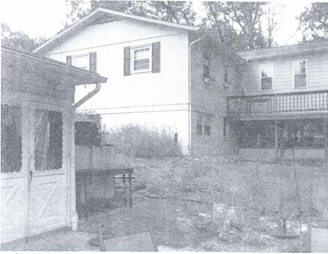
Left neighbor's house from left rear of 8210
